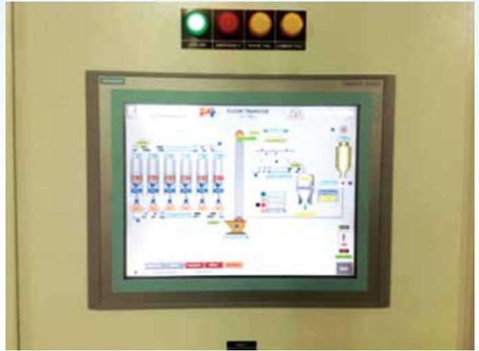
Flour Transfer System (HMI/SCADA view)
