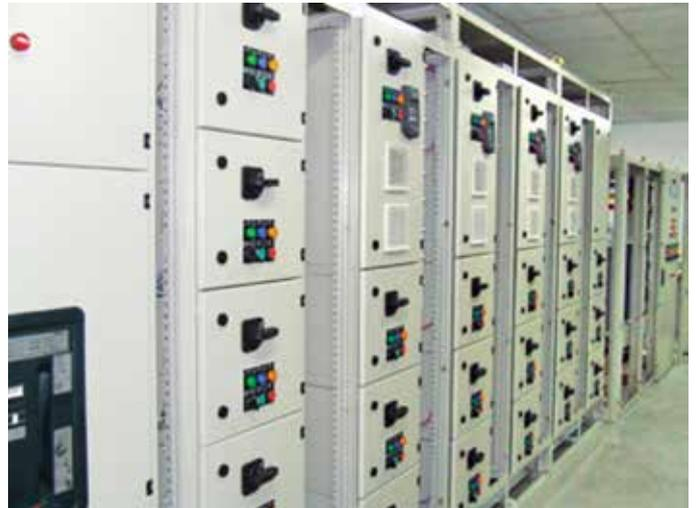
Fabrication of Electrical Panel FORM IV - MCC Panel (As per BS Standards)
